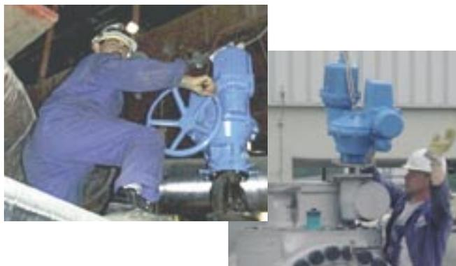
We offer the service of valve measuring, actuator sizing and mounting actuators by means of special adaptors to the existing valve interface. This kind of service has even to be considered strongly on automation and rehabilitation projects if for example the valve cannot be replaced from the pipe, long delivery times delay the project, or costs for a new valve plus actuator exceed the effect saved by the automation.
